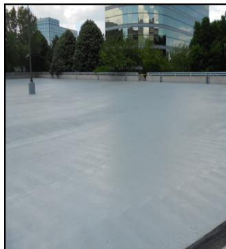
Traffic bearing deck coating prior to striping
