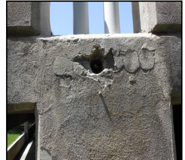
Evidence of Broken PT Cable
