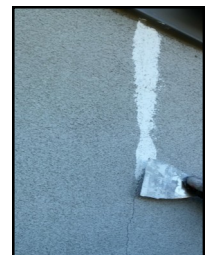
Patching facade prior to coating
