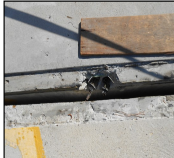
Broken Post Tension Cables
